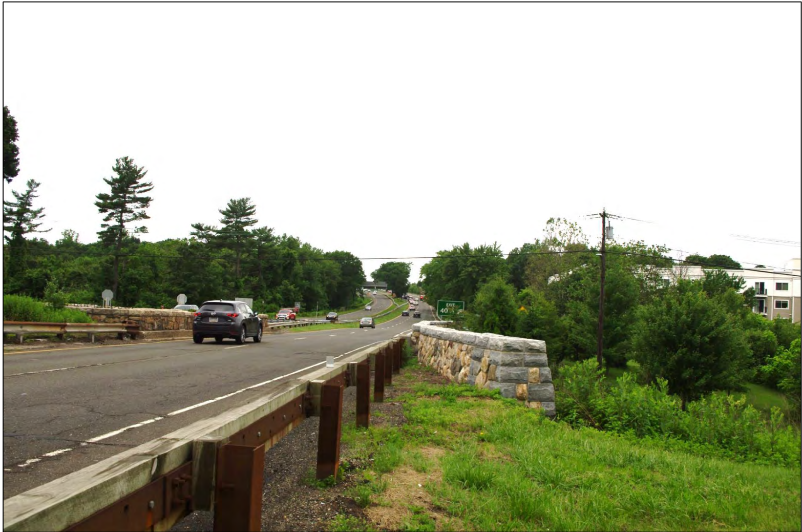
Photograph 31: Detail of the latest timber-on-metal guiderail, joining up with the parapets of the Main Avenue Bridge, camera facing southwest.
